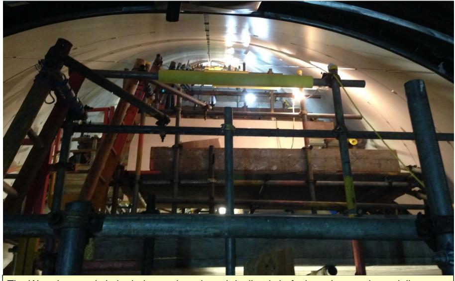
The Warerite panels in both the north and south inclined shafts have been substantially completed. Where the original panels had to be replaced panels have been provided by Formica whose predecessor supplied the original panels to the tunnels.
