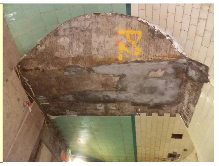
works. delaminated concrete in preparation for re-tiling The contractor has started to reinstate areas of
