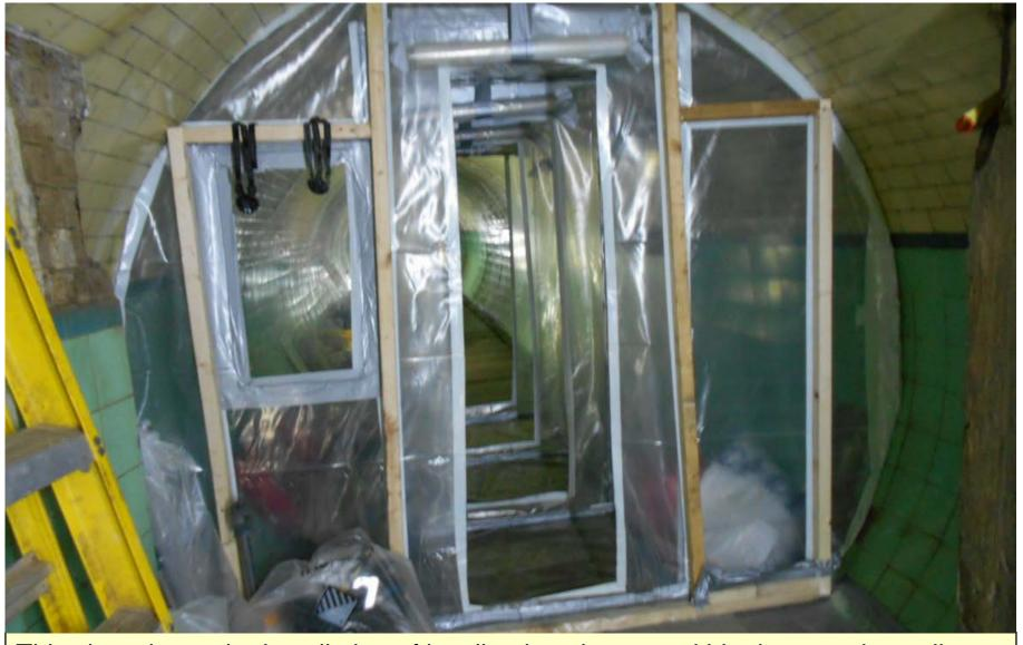
This view shows the installation of localised enclosures within the tunnels to allow specialist contractors to drill into the asbestos packing between the cast iron rings prior to the injection of resin to stop leaks.
