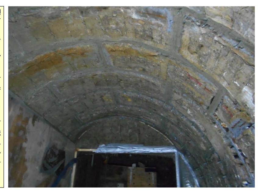
iron rings, which were leaking, have now been sealed. had all tiling removed and the joints between the cast The next operation waldecoe-tiling. This section of tunnel adjacent to the lift shafts has
