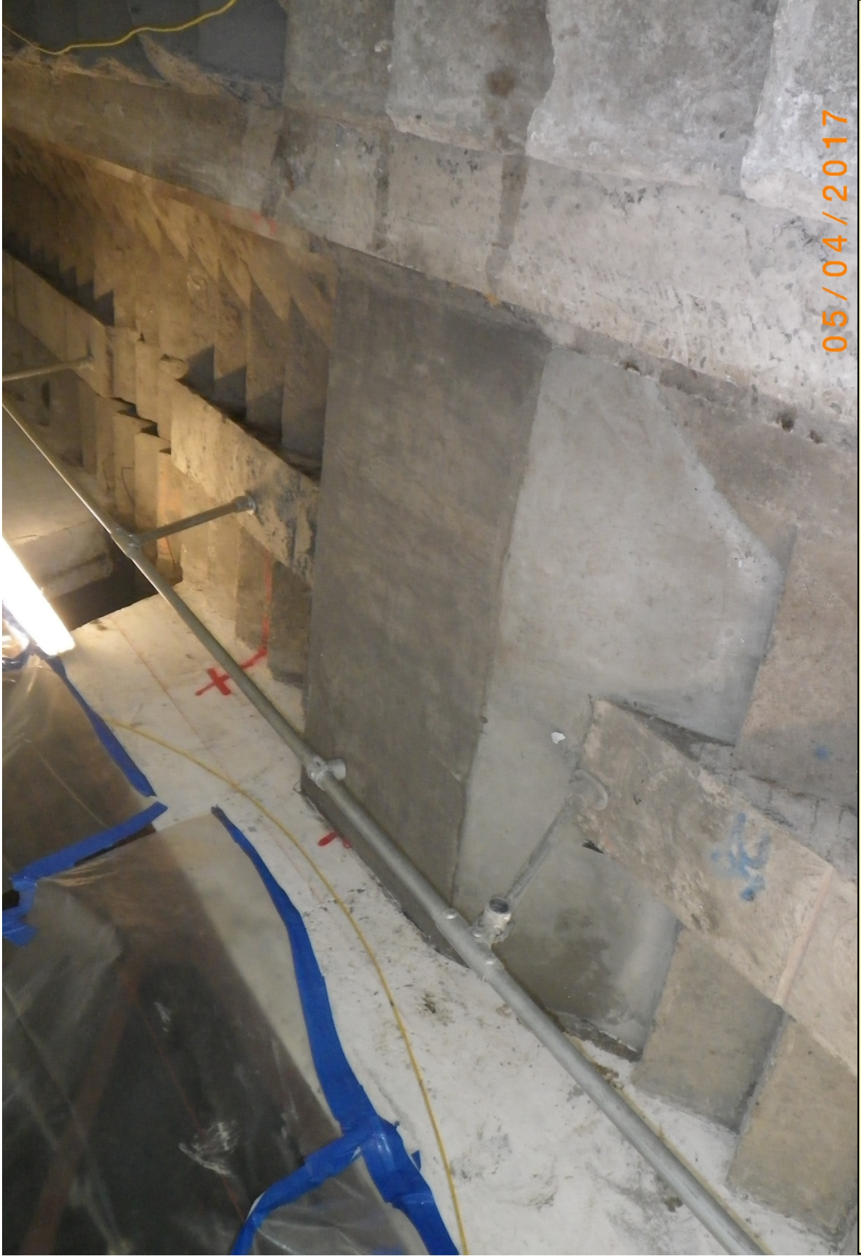
This view of the Jarrow inclined shaft shows the concrete plinths which have been constructed and will be used to support the guide rails for the new inclined glass lifts.
