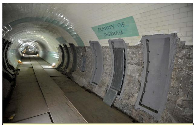
New ventilation ducts are being installed at the centre of the tunnels. Once these are complete the tilling can be replaced 76
