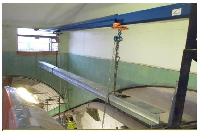
The steel rails which will carry the new inclined lift have to be lowered down the inclined shaft and fixed into position. Page 73
