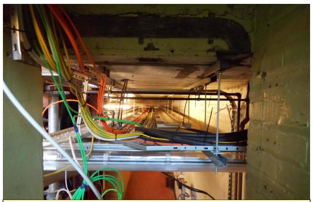
Thousands on metres of new cabling are being installed to service the lifts, lights, cctv and PA systems within the tunnels.
