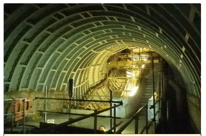
Once the original fabric, tiles and panelling, in the tunnel was removed leaks and corrosion repairs were carried out.
