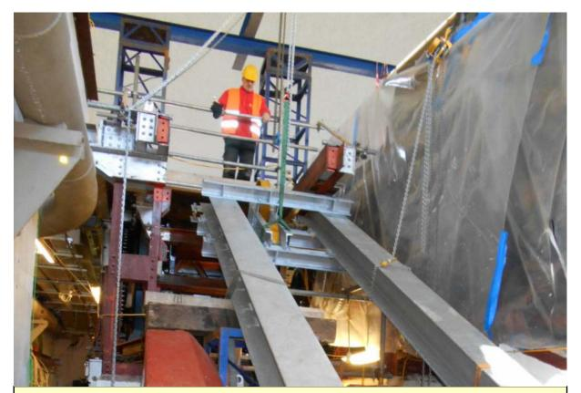
The rails to support the new inclined lift have been installed along with the motor and pulley wheels..
