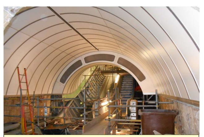
The lining panel system to the inclined shafts and lower landings have now been completed to replicate the original pearance of the tunnels.
