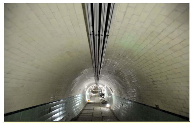
Tiling repairs to the crown of the tunnels have been completed and the trucking to carry all the new cabling, cctv, lights and PA equipment are being installed.
