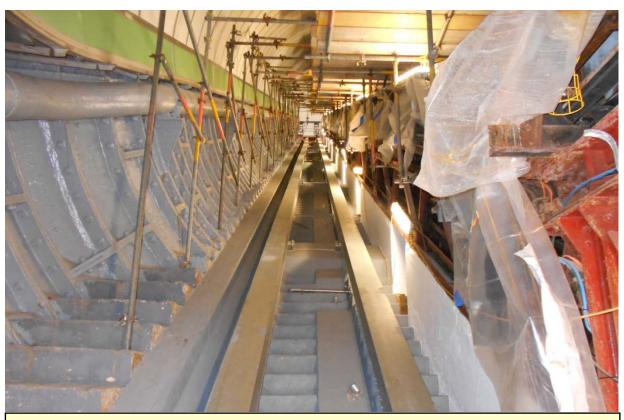
The rail track for the new inclined lifts have now been installed. The next operation will be to erect the lift car on to the rails.
