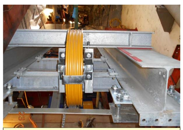
The pulley system used to lower and raise the new lift car has been installed. Page 75
