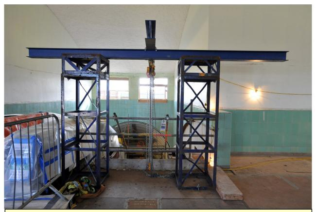
Specialist lifting equipment has been installed at the top of the inclined shafts to allow the installation of the new inclined lift to be carried out.
