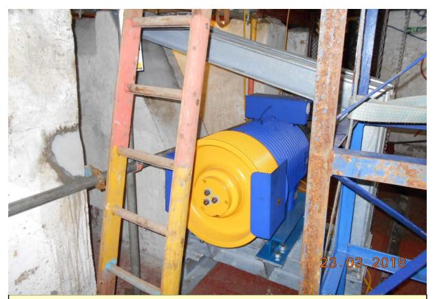
The motor required to operate the new inclined lifts has been installed. This will be wired up to the control panel and the lift car will be installed.
