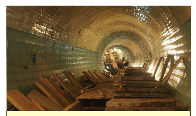
The tunnel paving has been lifted and relayed a number of times during the project to allow installation of new mechanical and electrical systems, to deal with structural repairs and asbestos removal.
