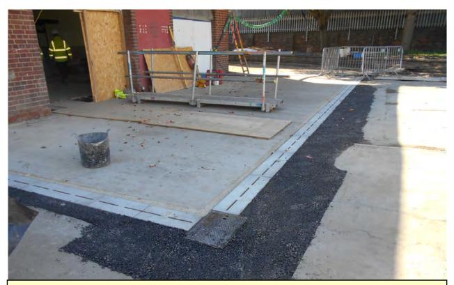
The concrete slab in from of the rotunda building has now been replaced as has the drainage. The next element of works attempt is the replacement of the surfacing.
